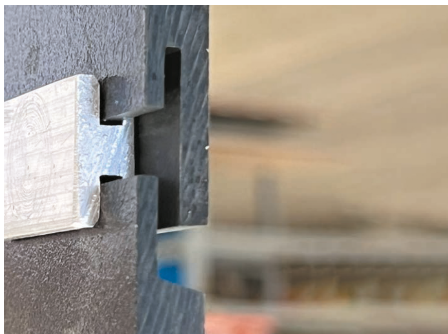
“Tongue & Groove” installation example
