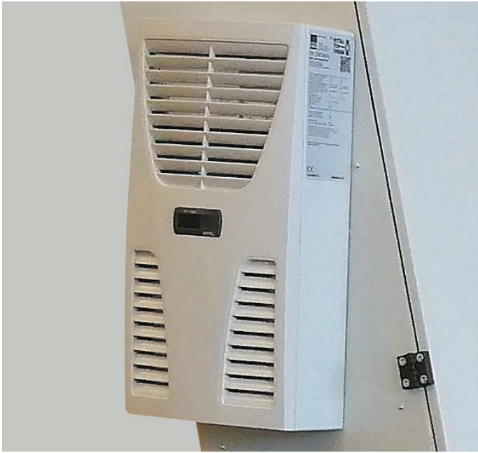
Cooling device for electric cabinet
